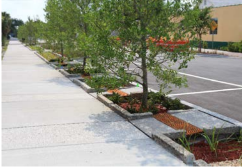
Infiltration pits can be integrated with formal street plantings
