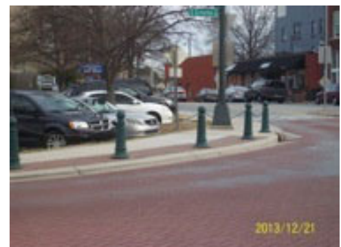
An example of bollards and chain being used to mitigate over-scaled curve radii
