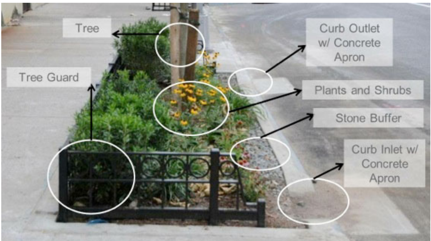
Examples of tree wells that function as water quality/management facilities (bio-swales), pedestrian safety features, & visual amenities
