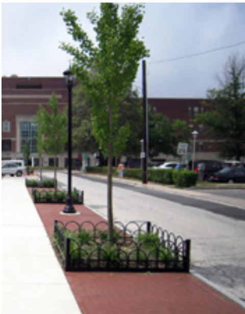
Pervious pavers over a covered soil area, an open soil area surrounding the tree, and a iron tree guard protecting the tree
