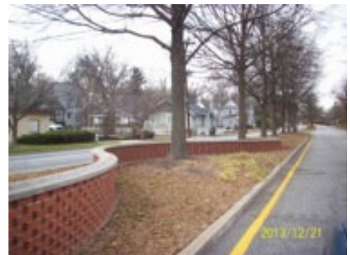
An example of a decorative wall that helps to protect street trees, while also serving as a traffic calming and pedestrian safety feature
