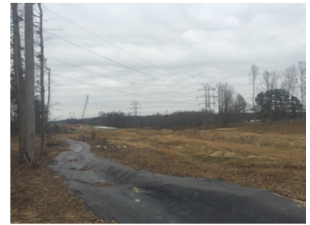
Urban Loop under construction at northeast corner of Keeley Park
